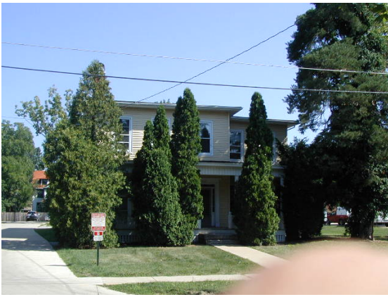
South Elevation – Before
