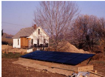
1.5 KwH adjustable PV array installed first to power tools
