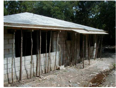
Constructing new housing
