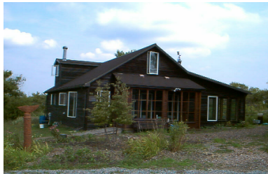
Macoskey Center west elevation
