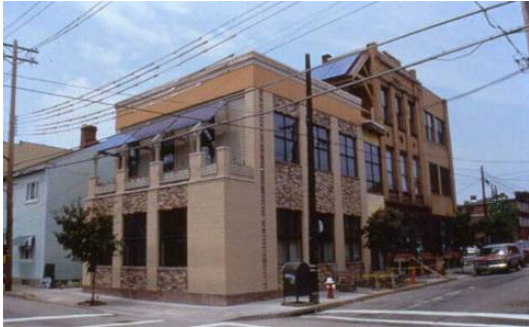
View from Southeast showing PV at porch
